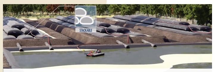
$\label{thm:containers} \mbox{Geotube dewatering containers can be stacked, saving valuable space.}$
